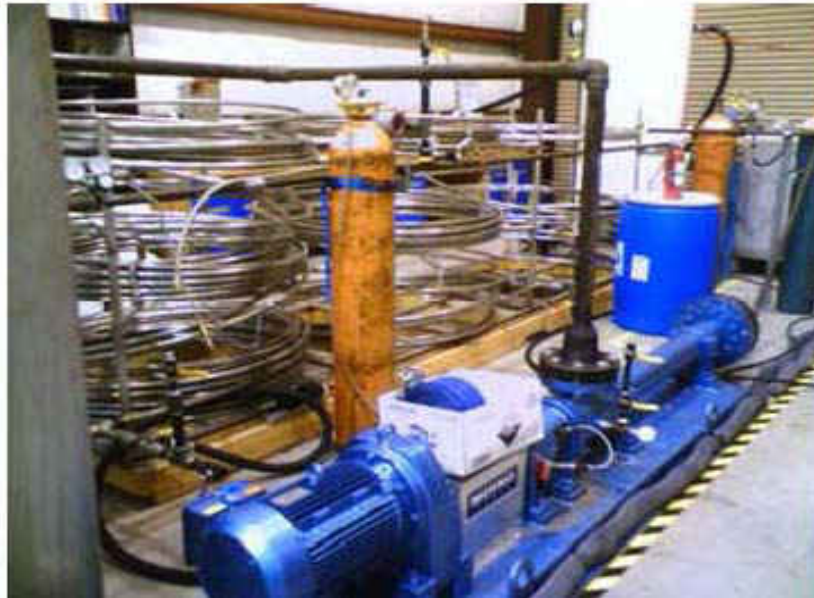
Figure 7: Completed scavenger system
